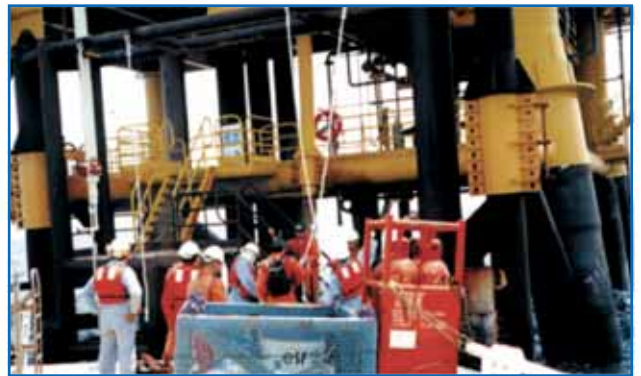
Installation Of FRP Grating On Offshore Platform (Brunei)
