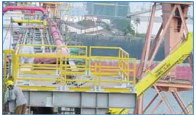
FRP Grating & Handrails For FPSO (Brazil)
